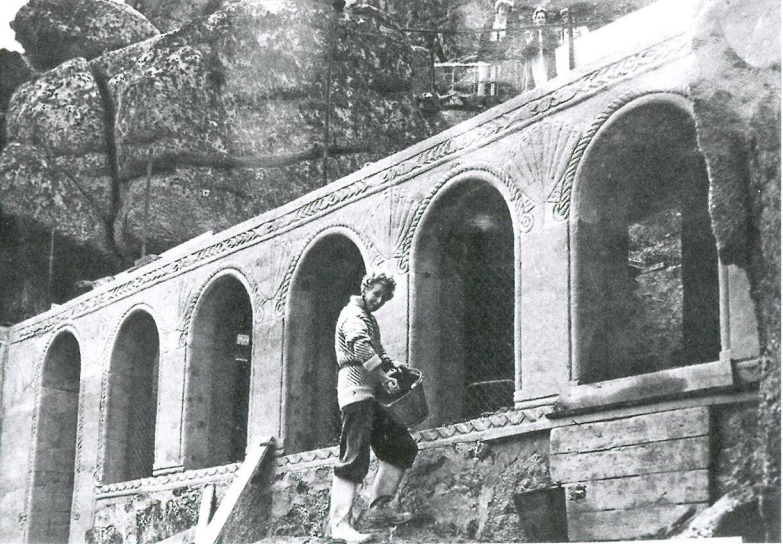
Rowena at work decorating the hand-built arches of the Minack's dressing rooms.
